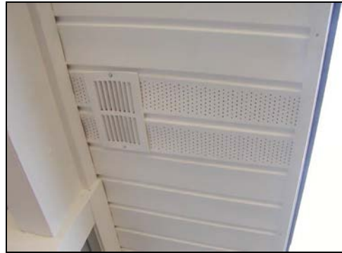
Figure D-1: At a minimum, outside air intake register mounted in vented vinyl soffit with OA duct positioned in soffit above.
