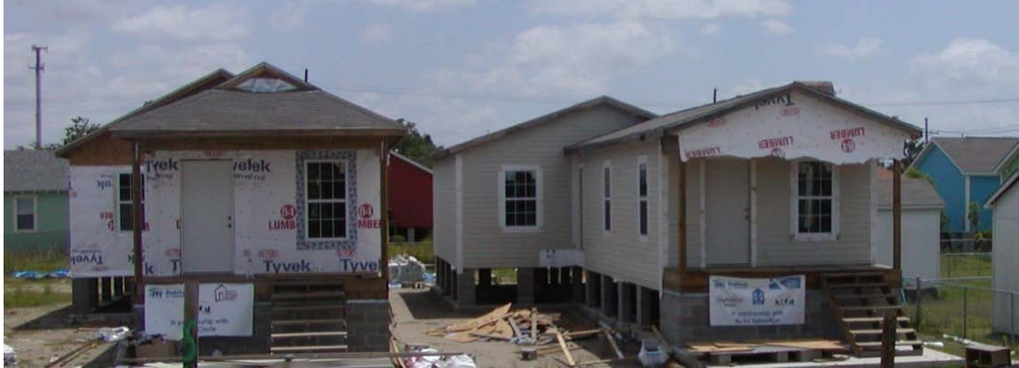
Figure 5. New Orleans Area Habitat 30% Prototypes – both failed the TBIC.
